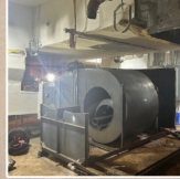
Old air handler system being demolished to make room for the new system
